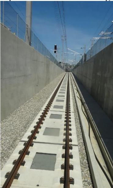
Figure 6 - Ballastless track in Vienna Central Station (Piereder, n.d.)
